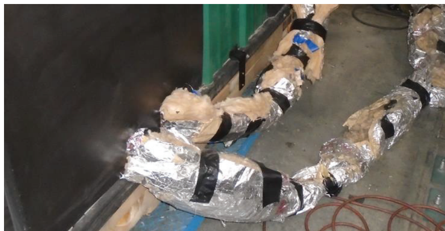
Figure 9 - Insulated Boiler Supply and Return Lines
