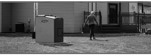
**Save Money & Fuel** - Heat buildings and water with the Maxim M255 PE outdoor wood pellet furnace. Electronic ignition saves fuel by stopping and adding fuel as needed.
