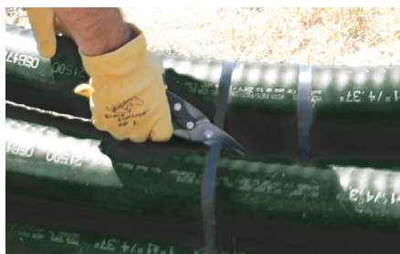
1 - Cut the three outermost fixing bands.
