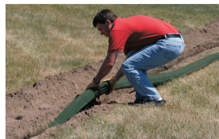
3 - Place ThermoPEX into trench.
