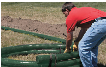
2 - Decoil to the next fixing band. Continue until decoiled.
